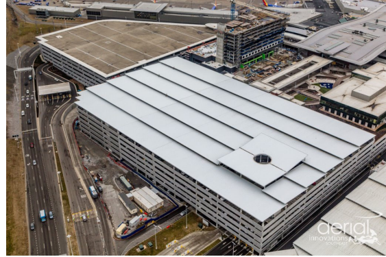
Opened Garage B
