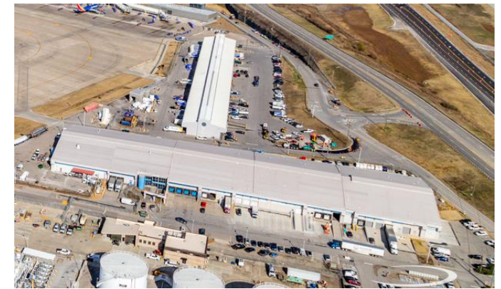
Multi-purpose/Air Freight Facility
