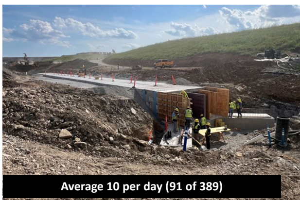
Block B-Center Box Culvert Installation, 9/3/25
