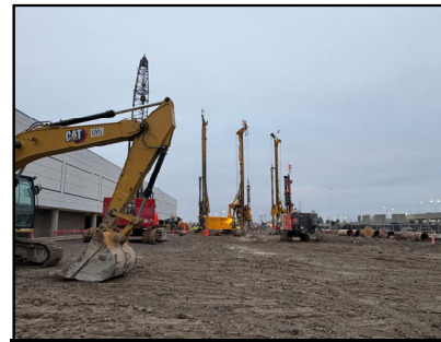
Drilled Foundations (24 of 280)
