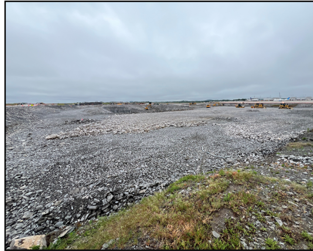
Central Ramp, May 7, 2026
