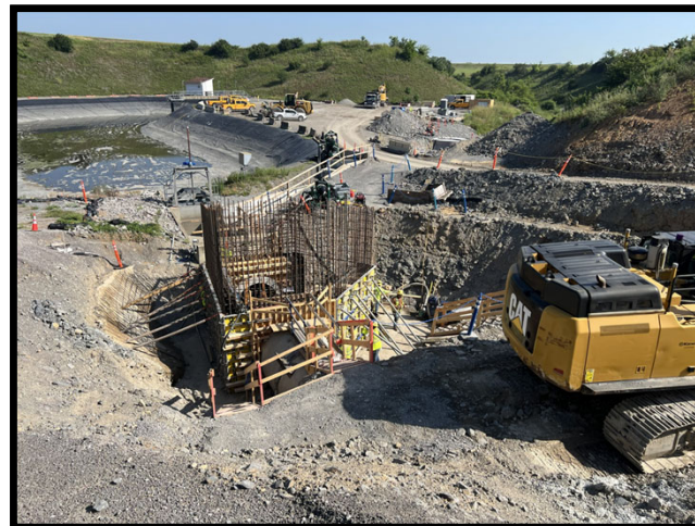
South Pond Diversion Structure, July 2, 2026
