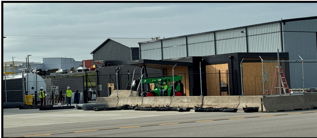
Jet Access AOA Fence Removal, July 6, 2026
